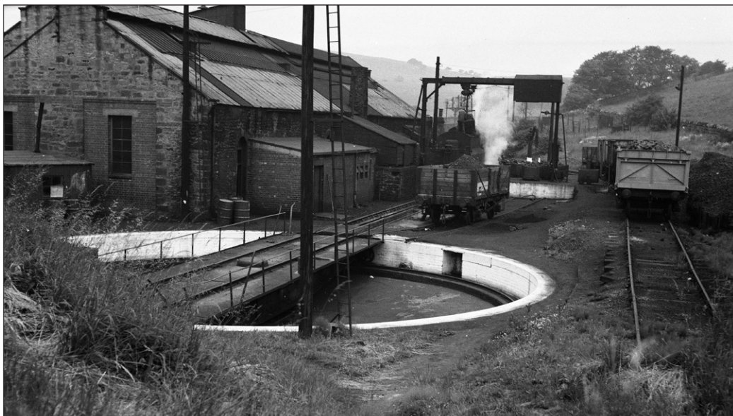
Above: A view of the original shed and 50ft turntable that was originally installed at Kirkby Stephen East MPD. The later electric coaling hoist is visible in the background. Fleetwood Shawe/SRC collection
